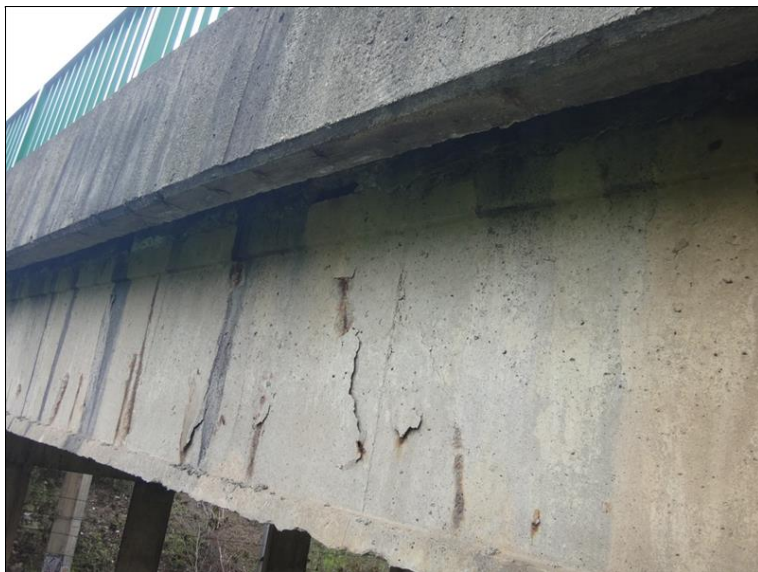
Detail čela NK s poruchami
